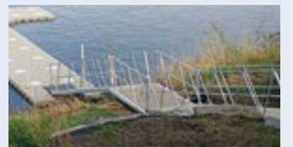
HANDRAIL INCREASES THE GANGWAY'S RIGIDITY AND SAFETY.
