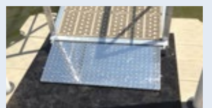
TRANSIT PLATE ENABLES EASIER ACCESS TO THE GANGWAY (WHEELCHAIRS, CARTS, ETC.).
